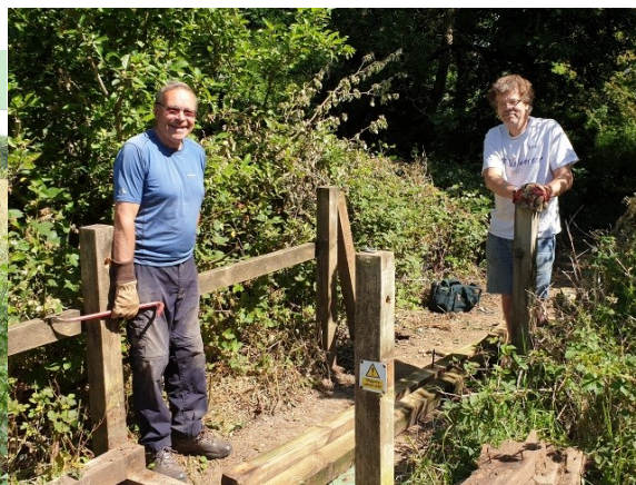
Dave and Peter working on the boardwalk
